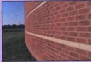
a brick wall / a wall made of bricks
